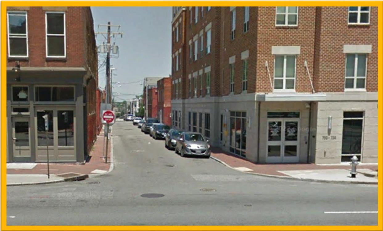
**Figure A-3: Missing Stop Bar and Crosswalk at Broad Street and Gilmer Street**
